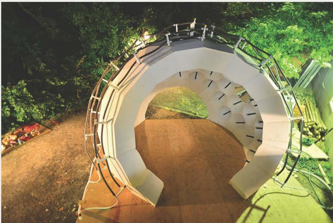
Thermoheliodome experimental reflective radiant cooling structure powered by indirect evaporation as part of the Beyond Shading project funded by the Andlinger
